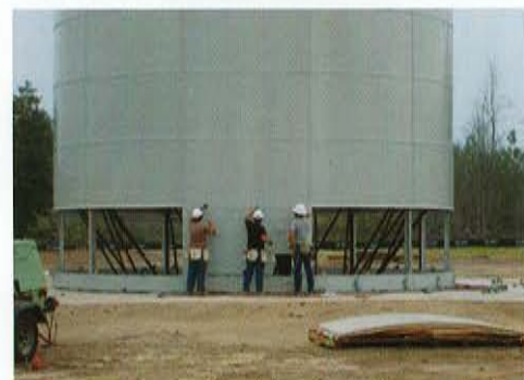
Standpipe - jacked from grade level
